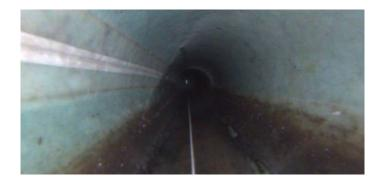
Code: Description: LFAC Lining Failure Abandoned Connection
