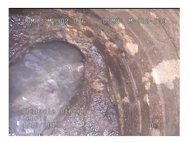
Code: OBZ Description: **Obstacle Other** Distance (ft): .0 Structural Grade: 0 O&M Grade: 5 Clock Start/From: 3 Clock To: 9 1st Value: 2nd Value: Value Percent: 40.000 Continuous Index: Within 8" of Joint: NO Remarks: debris
