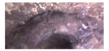
Code:JOLDescription:Joint Offset LargeDistance (ft):4.1Structural Grade:2O&M Grade:0Clock Start/From:0Clock To:11st Value:22nd Value:4Value Percent:1
