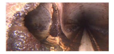
Code: TFD Description: Tap Factory Defective Distance (ft): 149.8 Structural Grade: 0
