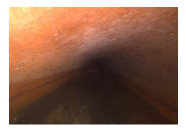
Code: MSA Description: Abandoned Survey Distance (ft): 39.4 Structural Grade: 0 O&M Grade: 0 Clock Start/From: Clock To: 1st Value: 2nd Value: Value Percent: Continuous Index: Within 8" of Joint: NO Remarks: **Possible Debris**
