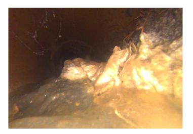
Code: OBZ Description: **Obstacle Other** Distance (ft): .0 Structural Grade: 0 O&M Grade: 4 Clock Start/From: 3 Clock To: 6 1st Value: 2nd Value: 30.000 Value Percent: Continuous Index: Within 8" of Joint: NO Remarks: **Mixed Materials**
