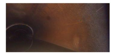
Code: Description: CL Crack Longitudinal
