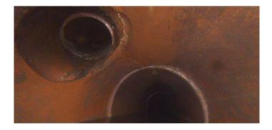
Code: TFD **Tap Factory Defective** Description: Distance (ft): 10.2 Structural Grade: 0 O&M Grade: 2 Clock Start/From: 11 Clock To: 1st Value: 4.000 2nd Value: Value Percent:
