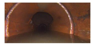
Code:FH2Description:Fracture Longitudinal Hinge, 2
