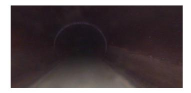
Distance (ft): 29.9 Structural Grade: 3 O&M Grade: 0 Clock Start/From: 3 Clock To: 1st Value: 4.000 2nd Value: Value Percent: Continuous Index: Within 8" of Joint: Remarks:
