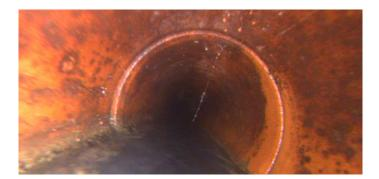
Distance (ft): 2.7 Structural Grade: 0 O&M Grade: 1 Clock Start/From: 1
