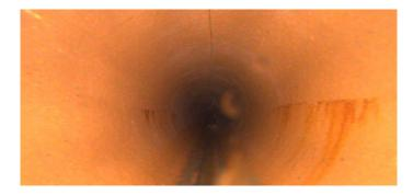
Code:CH3Description:Crack Longitudinal Hinge, 3
