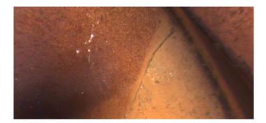
Distance (ft): 8.7 Structural Grade: 1 O&M Grade: 0 Clock Start/From: 2 Clock To: 3
