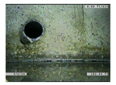
Code: JOMD Description: Joint Offset Medium Defective Distance (ft): 182.4 Structural Grade: 3 O&M Grade: 0 Clock Start/From: Clock To: 1st Value: 2nd Value: Value Percent: Continuous Index: F03 Within 8" of Joint: NO
