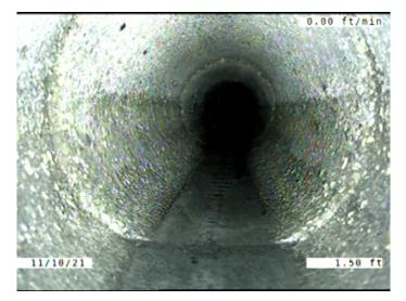
Code: MGO Description: **Miscellaneous General Observation** Distance (ft): 1.5 Structural Grade: 0 O&M Grade: 0 Clock Start/From: Clock To: 1st Value: 2nd Value: Value Percent: Continuous Index: Within 8" of Joint: NO Remarks: DROP INTO THE MANHOLE. HAD TO START IN THE PIPE.
