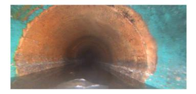
Code: MLC Description: Lining Change Distance (ft): 262.9 Structural Grade: 0 O&M Grade: 0 Clock Start/From: Clock To: 1st Value: 2nd Value: Value Percent: Continuous Index:
