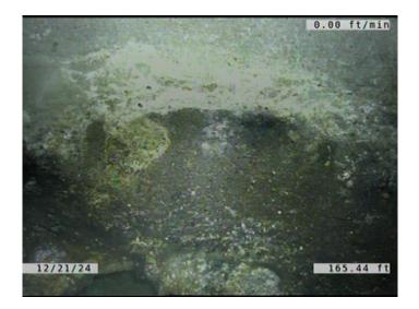
Code: MWLS Description: **Miscellaneous Water Level Sag** Distance (ft): 165.4 Structural Grade: 2 O&M Grade: 0 Clock Start/From: Clock To: 1st Value: 2nd Value: 10.000 Value Percent: Continuous Index: F06 Within 8" of Joint: NO
